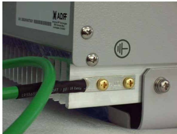
Figure 8 – Ground Cable Connection
